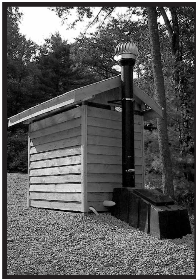
The Enviro Loo uses heat and air instead of water or chemicals to treat waste, and so does not threaten drinking water. The toilet also does not use electricity.
