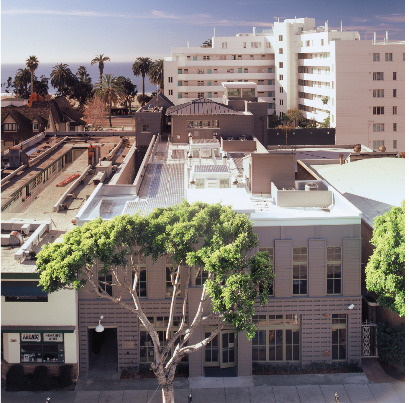
The NRDC's century-old frame belies the building's modern green renovations, which earned it a LEED platinum rating.
