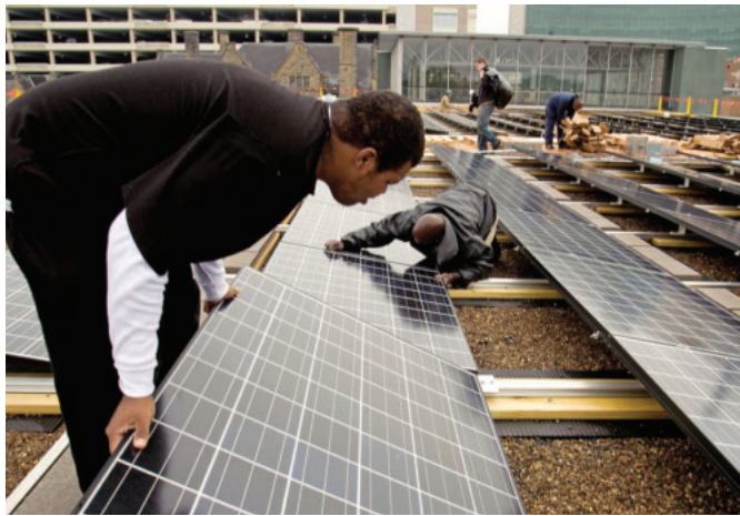
Ohio Cooperative Solar workers install solar panels atop a building on the campus of the Cleveland Clinic.
