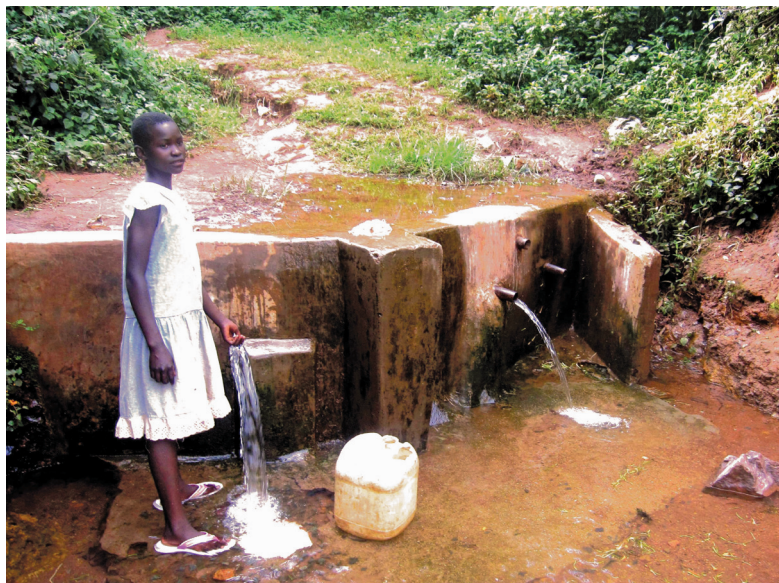
A girl in Kenya's Kisii District draws water from a local spring that has been protected through concrete sealing.
